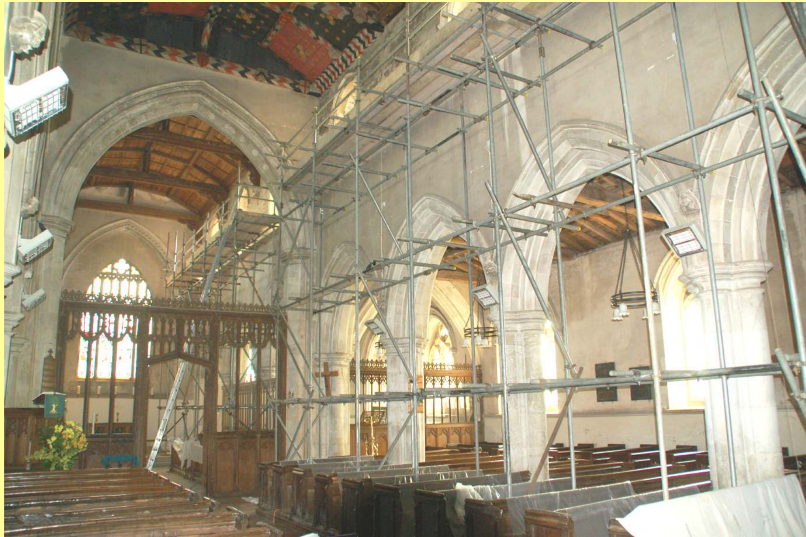
Scaffolding was erected to give access to the windows
