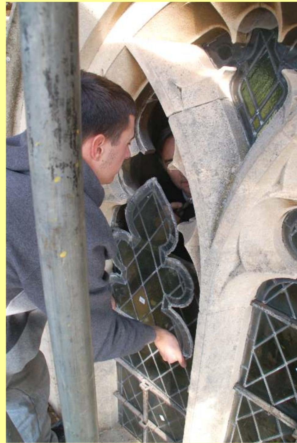
Each pane was removed from its frame and the ironwork removed for repair. The window openings were blocked off.
