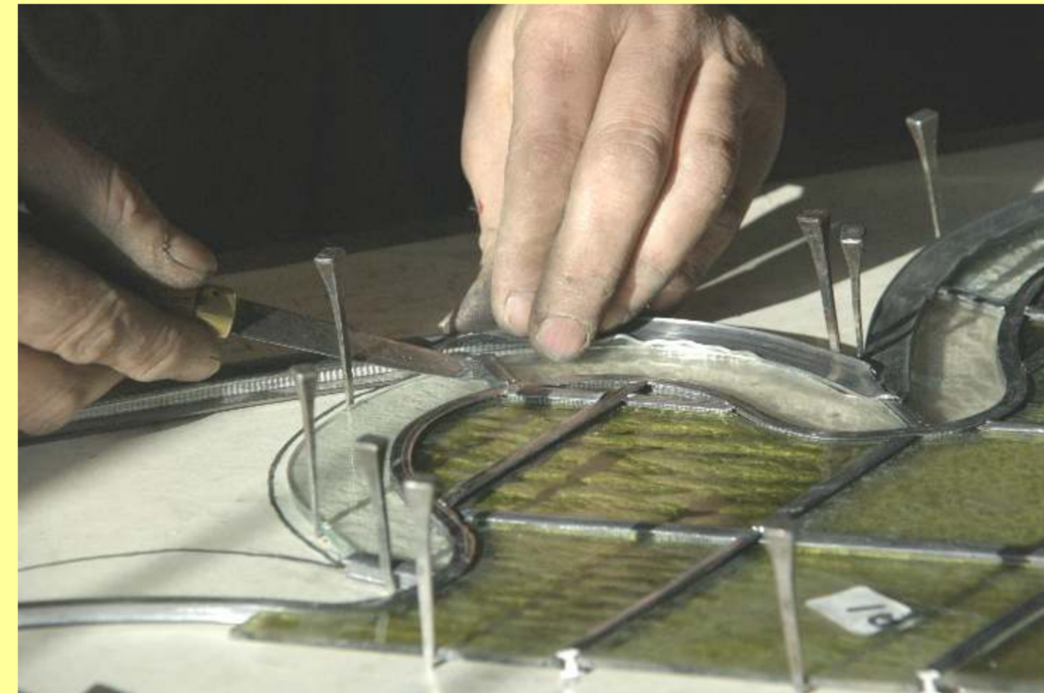
Each pane was taken apart and rebuilt using new leading. The new assembly was waterproofed and finished ready for re-installation.
