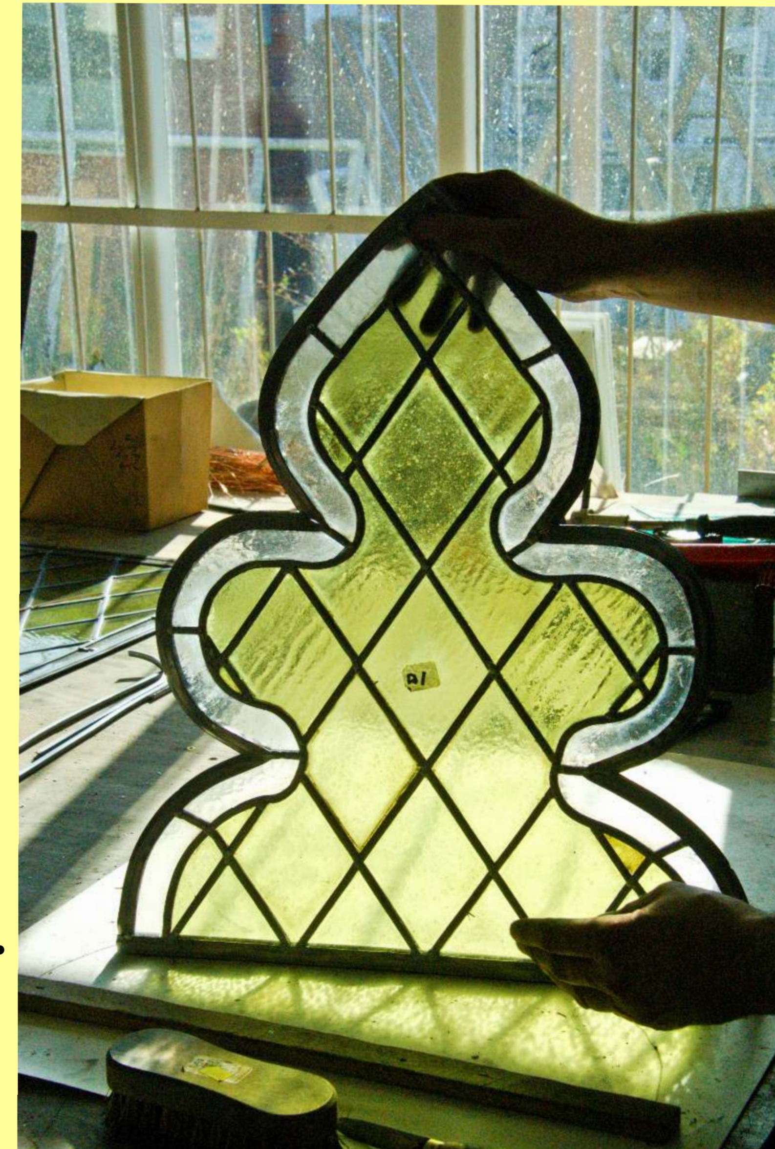
Each pane was removed from its frame and the ironwork removed for repair. The window openings were blocked off.
